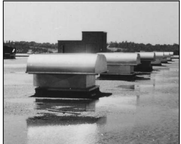
Hooded Propeller Roof Ventilator
