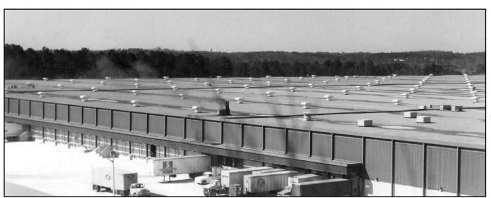
Hooded Propeller Roof Ventilator
